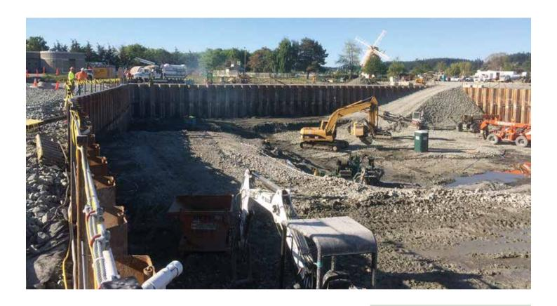
The City of Oak Harbor New Clean Water Facility project in Windjammer Park had a watertight seal requirement. Nucor Skyline supplied a sheet pile system designed to shore the surrounding site and cut off water for the new structure, which was 25' below grade in beach deposits.
